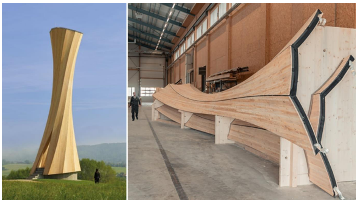
Fig. 3. Surface-active structure made of single-curved CLT components, Urbach Tower ICD/ITKE Research Pavillion, Stuttgart, 2010 (source: elaborated by M. Golański based on [5])
