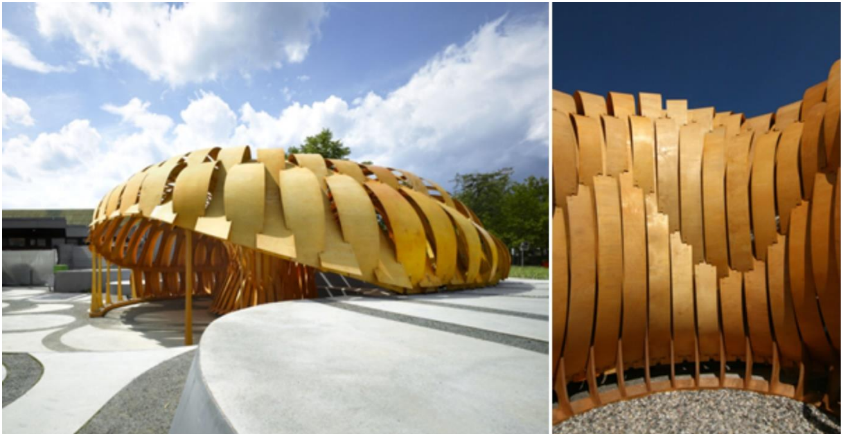
Fig. 2. Bending-active plate structure, ICD/ITKE Research Pavillion, Stuttgart, 2010 (source: elaborated by M. Golański based on [6])
