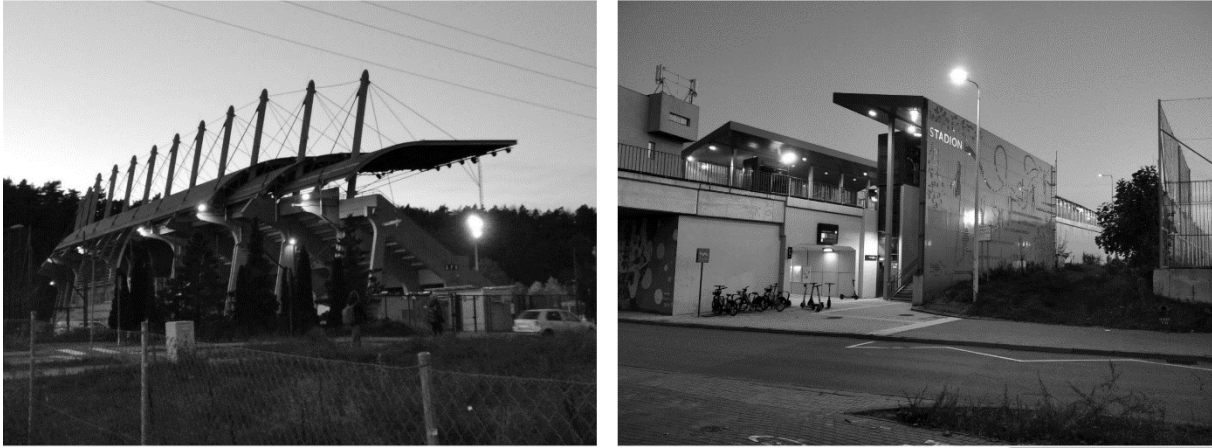
Fig. 7, Fig. 8 Hanging form of roofing for Rugby stands. Minimizing the coverage of the Gdynia Stadion suburban railway stop.
