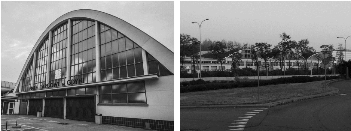
Fig. 1, Fig. 2. Paraboloid shapes on facades and roof structures of the Market Hall in Gdynia and the Pomeranian Science and Technology Park in Gdynia.
