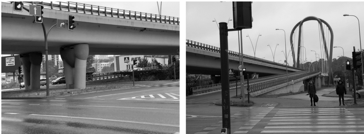
Fig. 9, Fig. 10. Searching for a sophisticated form of the pylon of the bridge over the Brda River in Bydgoszcz with a cable system. The supports and beams of this crossing with the bridge over the Brda in the area above one of the main road intersections have a completely different character.
