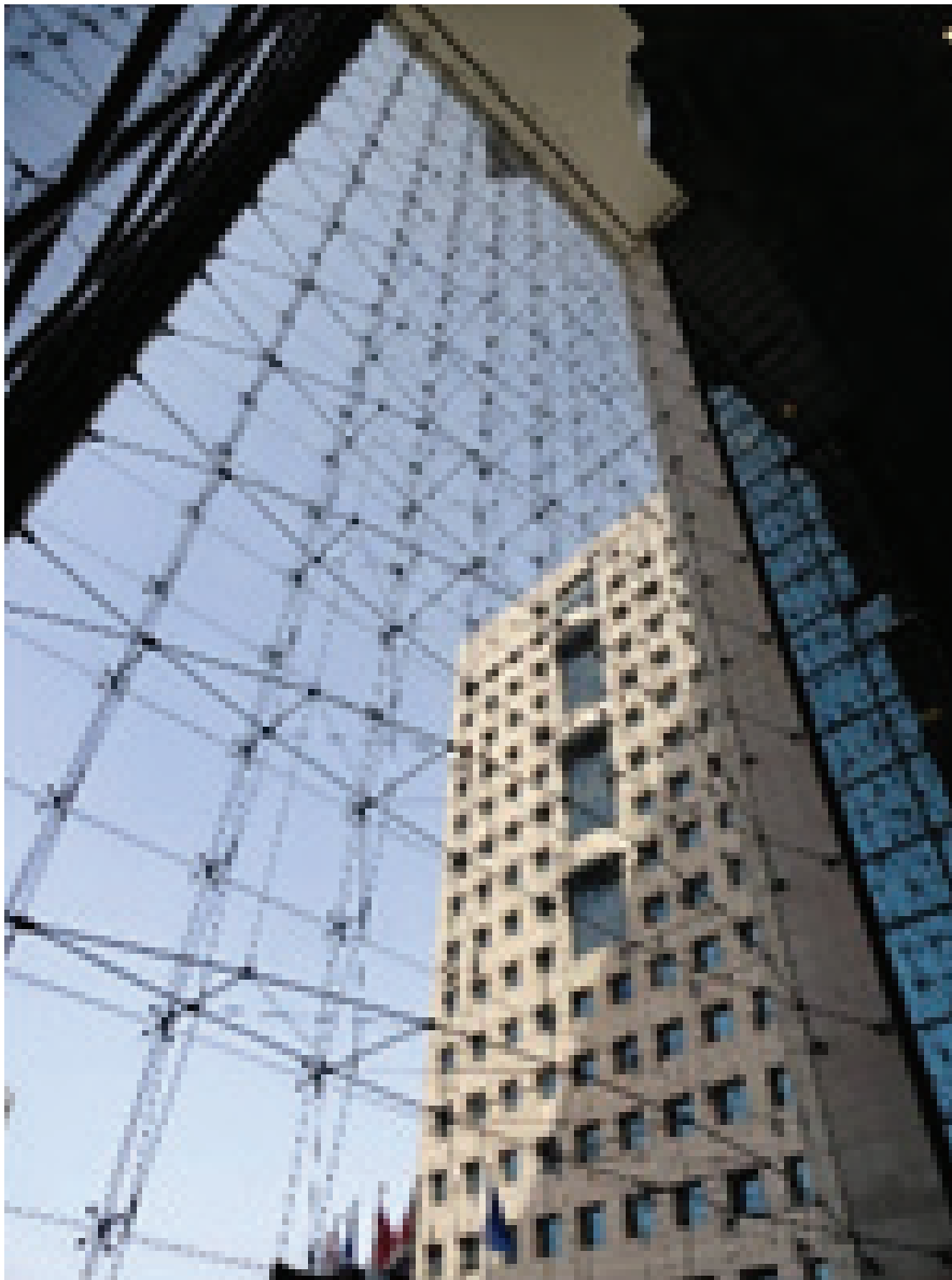
Fig. 8. Tensegrity glass facade, 1991
